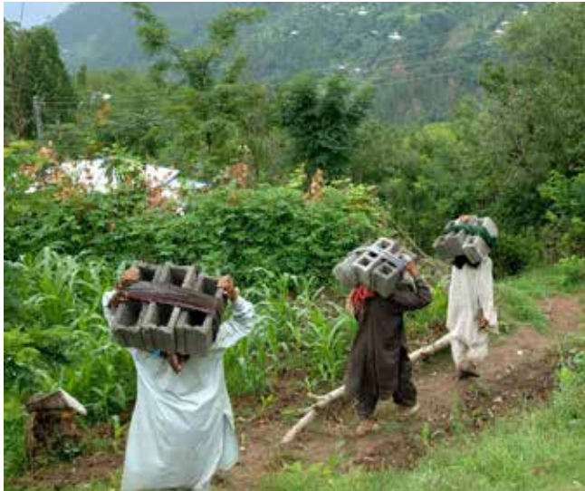
Remote communities had to summon all possible means to transport construction materials to building sites.
